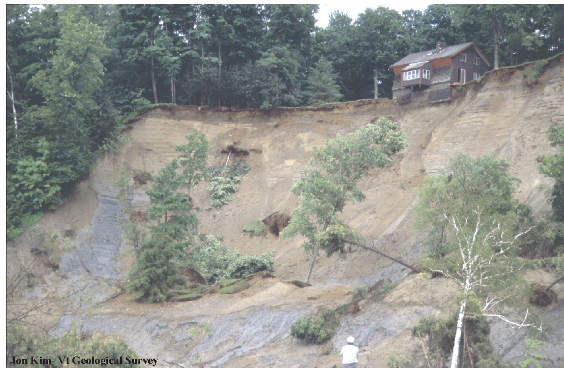
Figure 1. Photograph of the landslide site at DRH following the 1999 event (VGS 2018).
