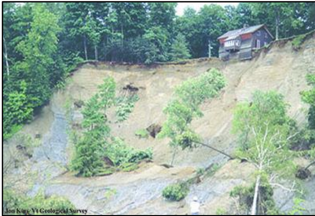
Figure 2. The Jeffersonville landslide site after the event in 1999, showing the overhanging home (Vermont Geological Survey, 2018).
