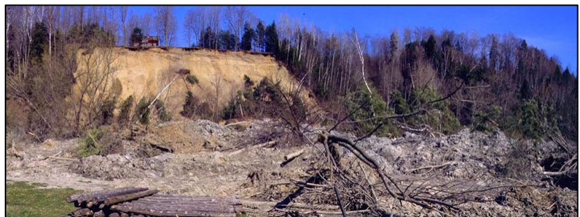
Figure 1. The landslide site showing the debris (Vermont Geological Survey, 2018).
